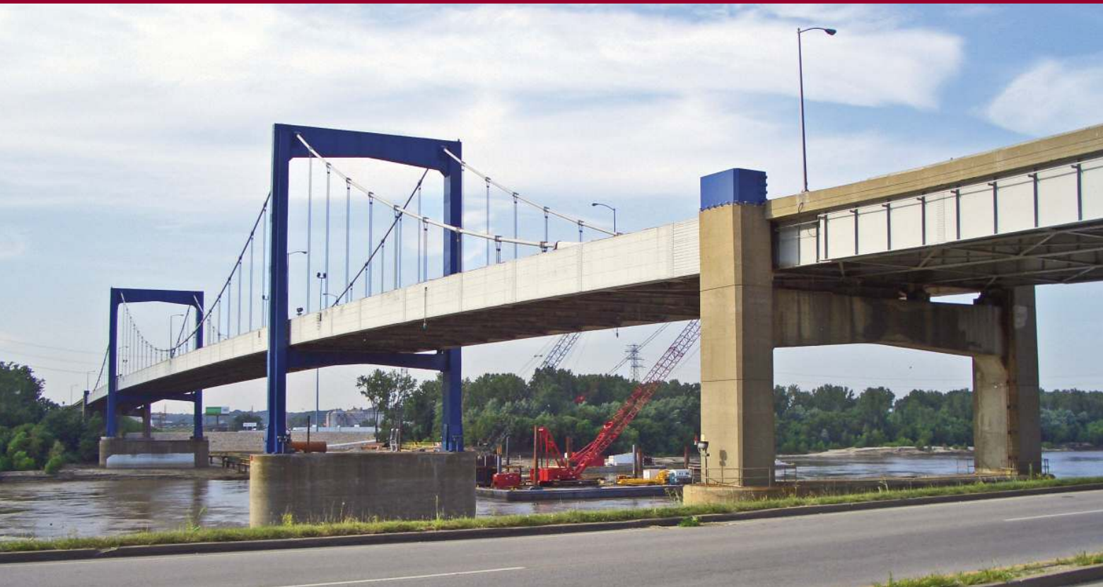
Figure 1. The old Paseo River Bridge before construction.
