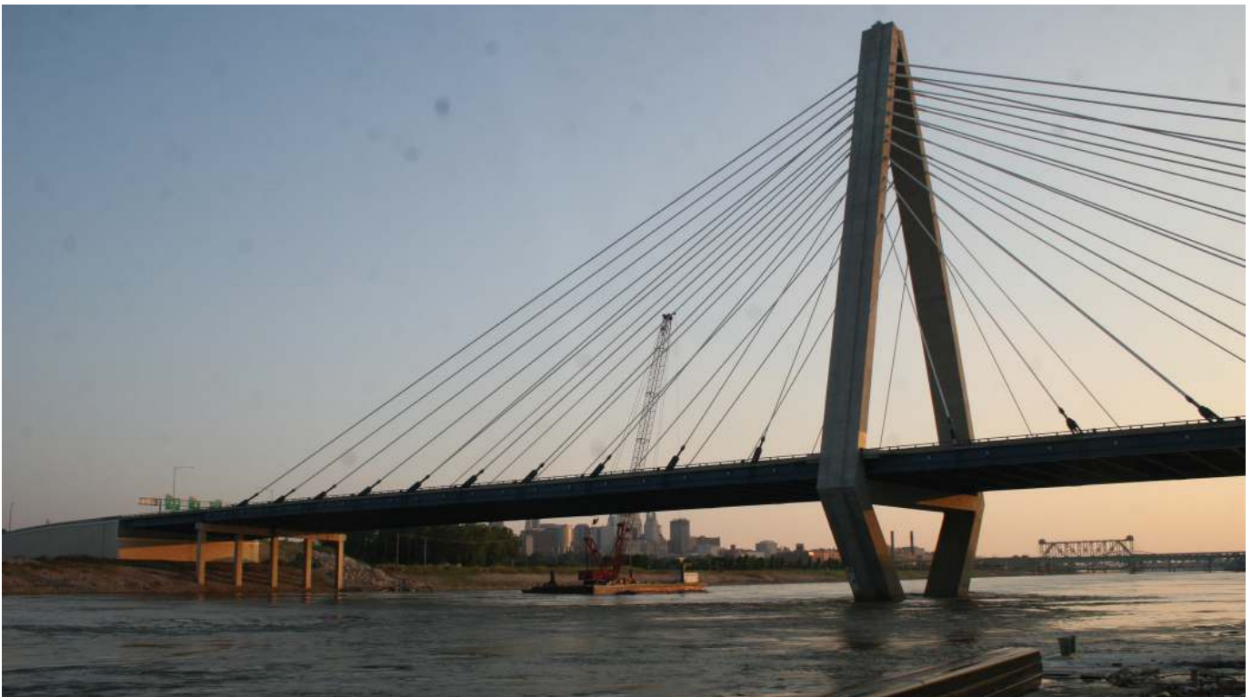
Figure 9. The new Christopher S. Bond Bridge.
