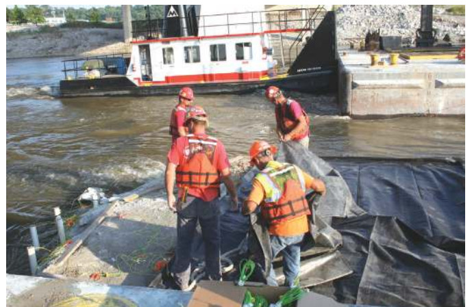
Figure 7. Placing the geotechnical fabric.
