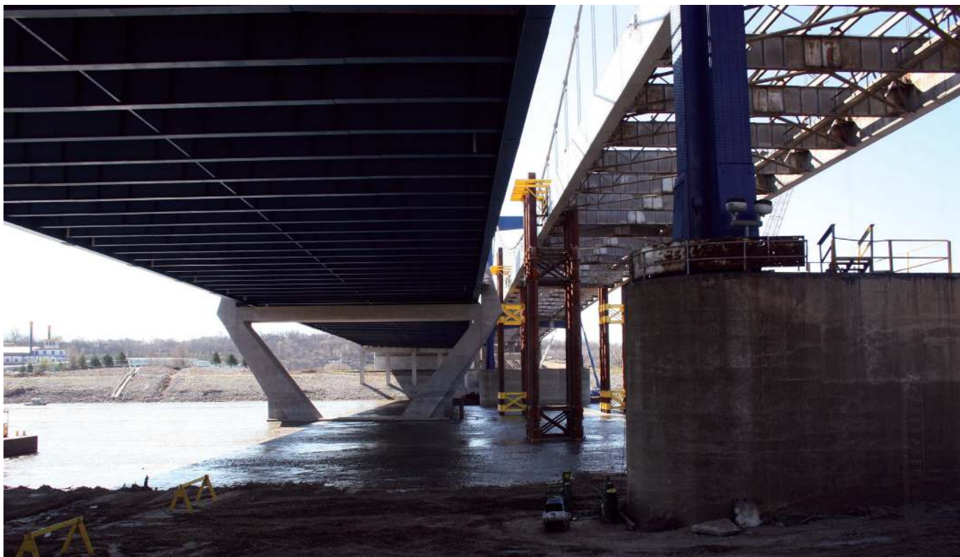
Figure 2. The old Paseo Bridge and new Christopher S. Bond bridge, before the old bridge was taken down.
